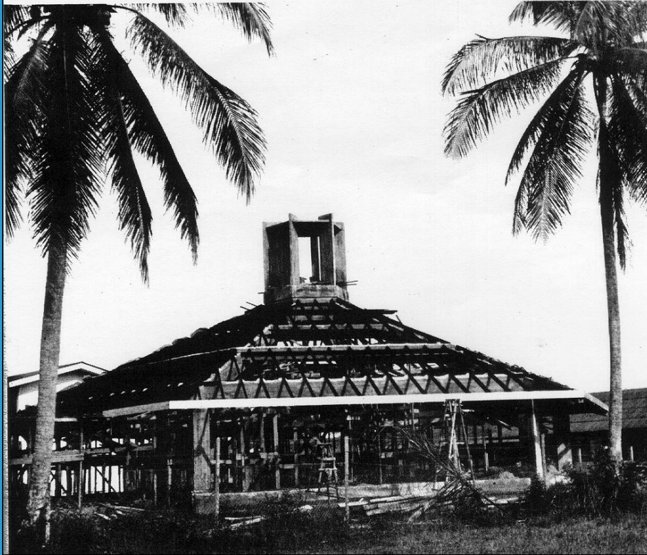
1971 - The new St. John's Church under construction.
